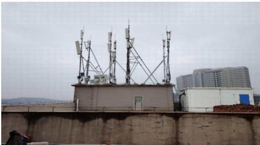
Figure 6.3. Application Case of Intelligent Power Distribution Unit with Extreme Energy Saving
